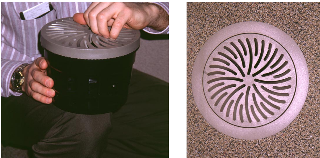
Figure 3. The Owens Corning headquarters building features an underfloor air plenum with Titus™ swirl-plate diffusers providing a flow rate between 0 and 90 cfm each.
